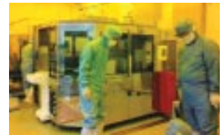
Installing state-of-the-art equipment
