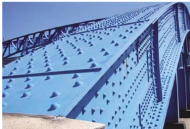
Fig. 1 Rivet structure for the Komagata Bridge in Asakusa
